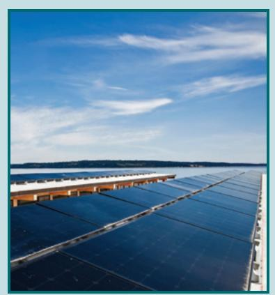
Thanks to a generous lead gift from the Martin-Fabert Foundation and the good work at Power Trip Energy, the Northwest Maritime Center now boasts a 24kw solar panel array on the roof of the Weissblum Maritime Heritage Building. In total, the new panels will produce more than 10% of the power needed for the building, with room remaining to add panels and increase our usage of clean, sustainable energy.
