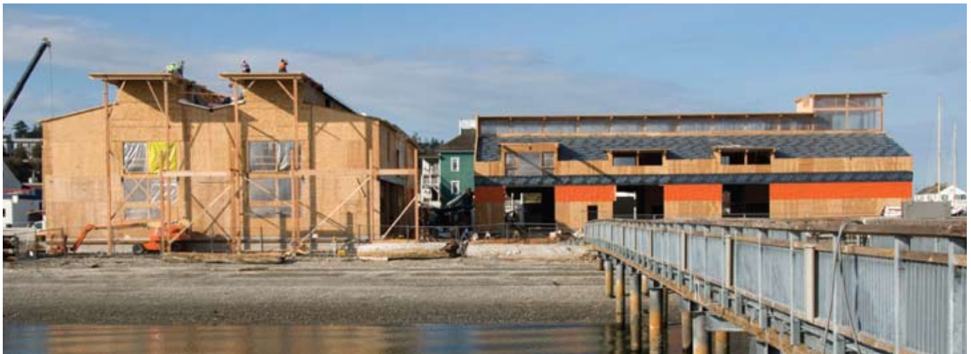
bottom: Northwest Maritime Center construction progress as of February 20, 2009.
